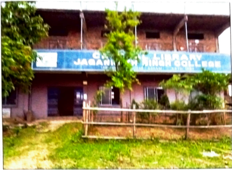
Front view of Library Building
